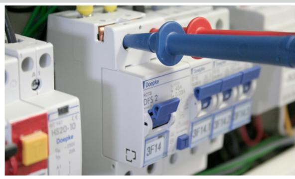
It is recommended that great care is taken when testing residual current circuit-breakers. Different factors need to be taken into account depending on the device type.
